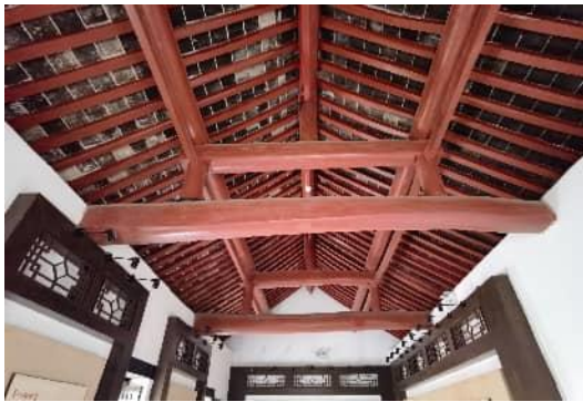
Figure 4. Timber structural frame.
